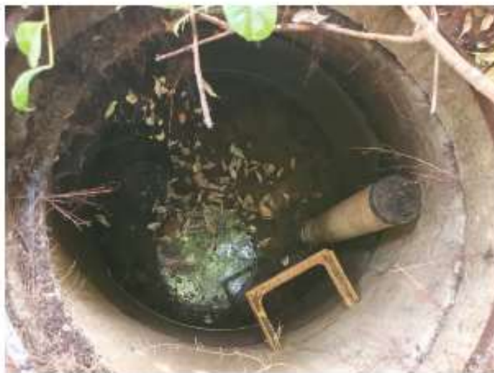
Image 2 – SW Pit 45, unable to visually inspect and measure pipes. Pit is full of water and has sealed plumbing features below the water line
