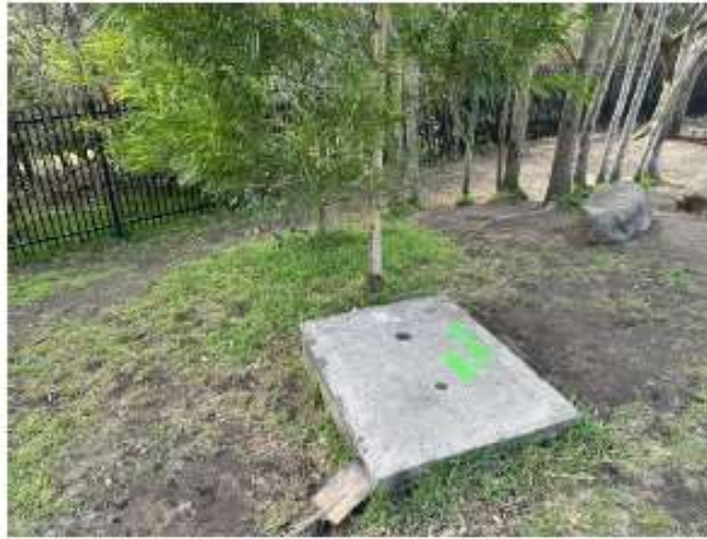
Image 3 – SW32, Stormwater pit cover that cannot be manually lifted by a two-person team 300kg +. The lip fitting prevents the lid from being able to slide off for inspection- mechanical lift required for inspection.
